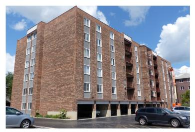
The Diplomat of Des Plaines Condominium Building is a 6-story residential community constructed in the mid-1970s. The building consists of 43 residential condominium units. The exterior walls consist of brick masonry cladding over concrete masonry unit (CMU) back-up wall. Cement board cladding panels are located at the floor lines between the windows.
